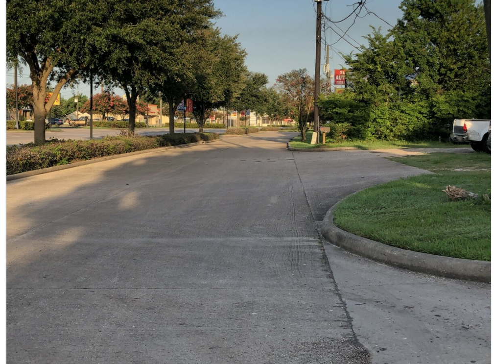
View of large apron access to S. Main
