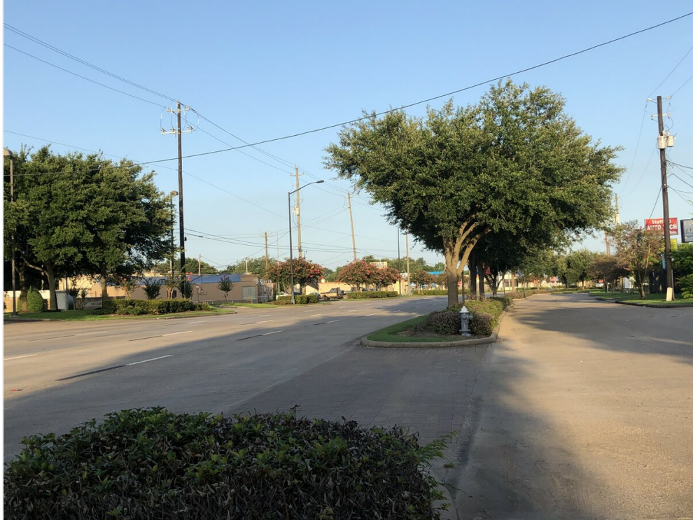
View of S. Main & Access road
